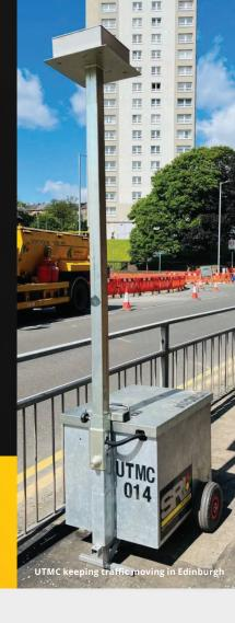
"The ability to combine the flexibility of using temporary signals whilst also being able to control and co-ordinate timings with the Council's existing permanent traffic signals, has been invaluable during construction works on the Trams to Newhaven project. Having now experienced the advantages of using the UTMC temporary signals, we will be looking to specify their use in future projects to help keep everyone moving around Edinburgh as the city builds for a brighter, greener future."
