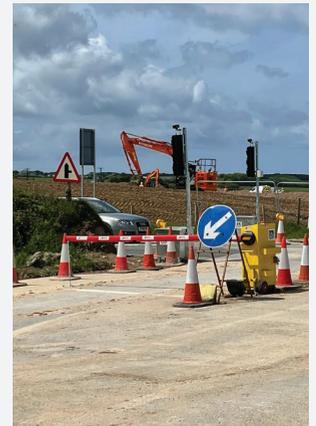
Haul Route PLUS automatically switches between the main road and haul route barrier system through detection of haul route plant vehicles. This is a wholly wireless process which prevents the need for manual activation.
